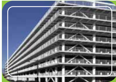
Multi-storied Steel Building
